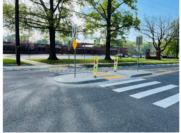
Figure 17 - New pedestrian refuge island at Wood Middle School.
