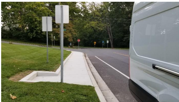
Figure 27 – New sidewalk to bus stop at Kensington Pkwy and Bexhill Drive.
