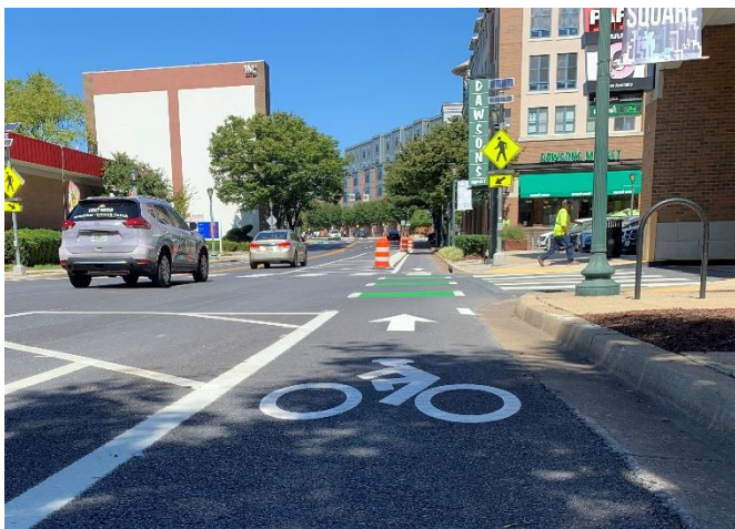
Figure 9 - City of Rockville installing protected bike lane along North Washington Street summer 2023.
