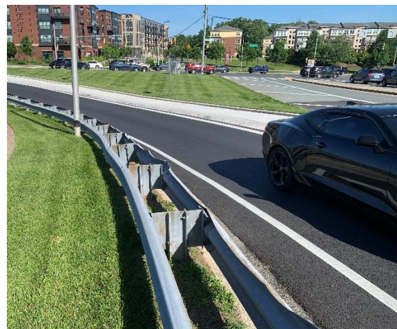
Figure 10 – Narrowed right turn lane to reduce right turn speed from Sam Eig Hwy to Diamondback Dr.
