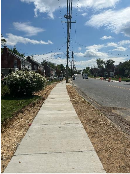
Figure 14 – Completed sidewalk along Oakview Drive.
