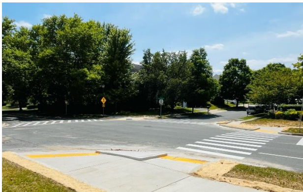
Figure 15 – New ramps and high visibility crosswalks in the Dr. Sally K. Ride Elementary walk shed.
