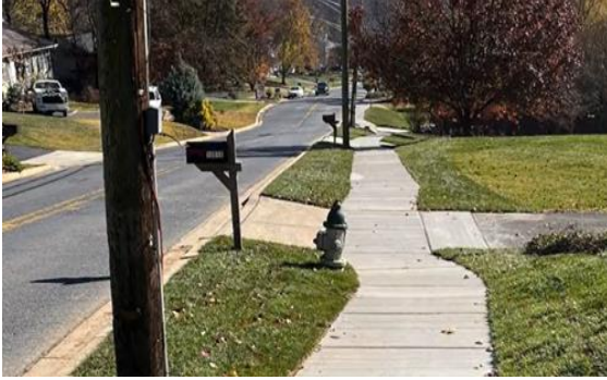
Figure 20 – Completed sidewalk extension project along the south side of Sweepstakes Road in Damascus.
