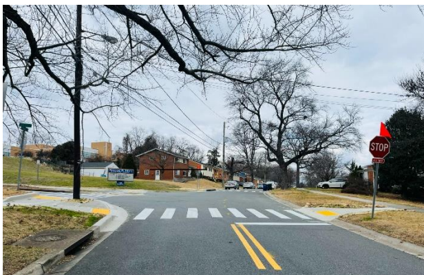
Figure 16 - New crosswalk and all way stop installed in Roscoe Nix Elementary walk shed.
