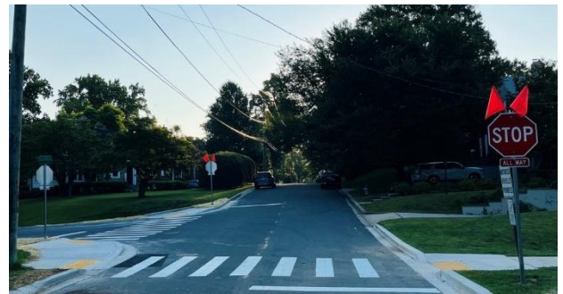
Figure 18 - All way stop, new ramps, and crosswalks at Cherry Tree Lane and Hillmoor Drive in Blair High and Pine Crest Elementary walk sheds.
