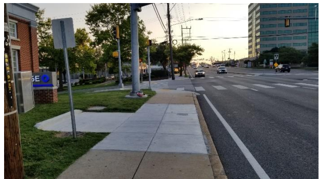
Figure 28 – Sidewalk repair and additional pad at University Boulevard and East Avenue.
