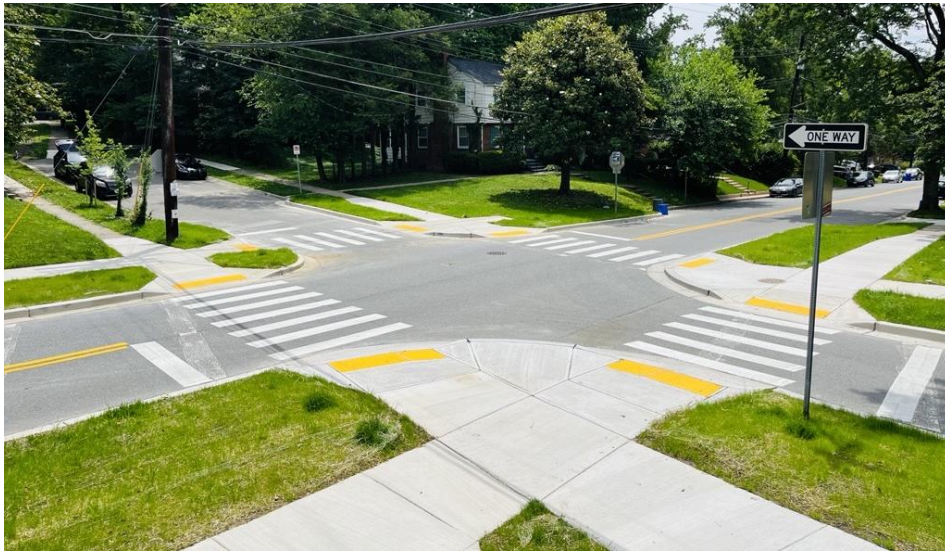
Figure 18 - Intersection narrowing and straightened crosswalks at Sundale Drive and Quinton Road near Rosemary Hills Elementary.
