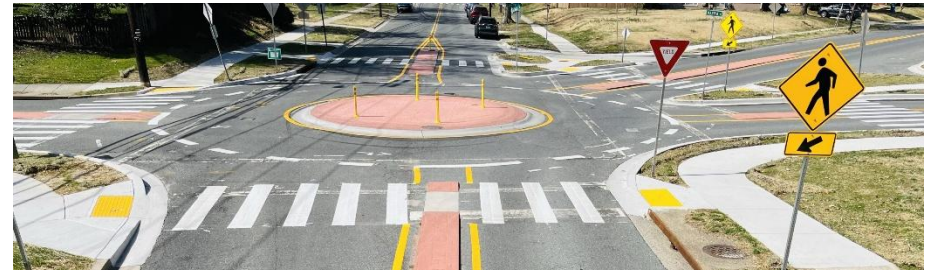
Figure 20 - Conversion of intersection of Dennis Avenue, Edgewood Avenue, Marvin Road to a roundabout.
