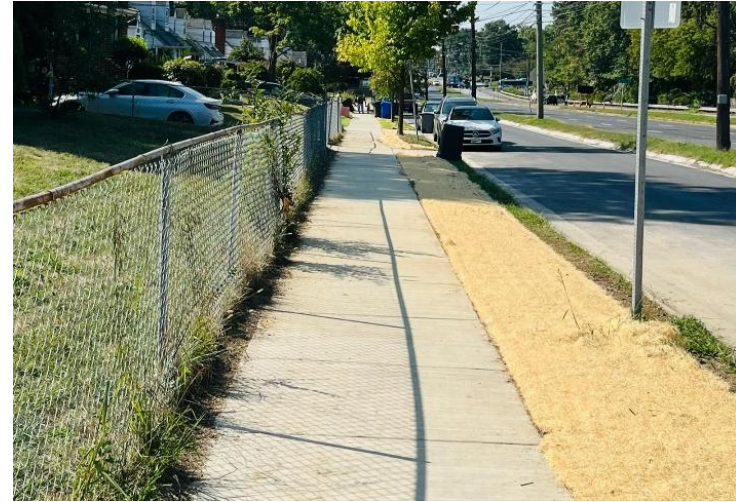
Figure 12 - New sidewalk installed with grass buffer on New Hampshire Avenue Service Road.
