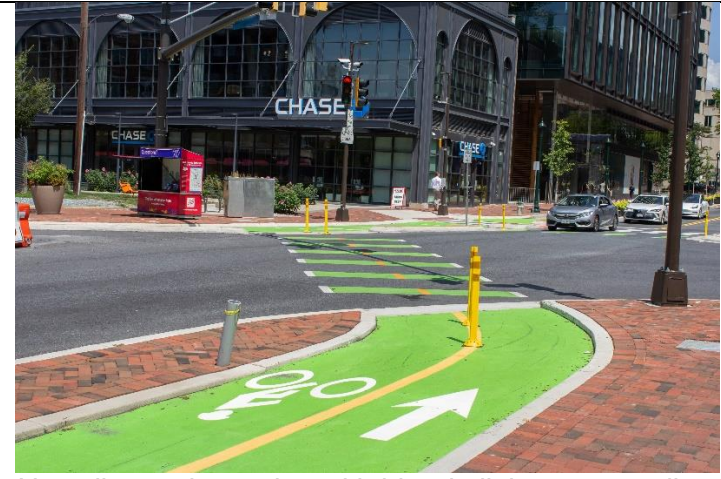
New diagonal crossing with bicycle light to get cyclists across the Bethesda Ave & Woodmont Ave intersection.
