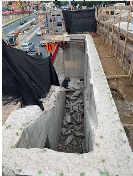
Demolition work for Metropolitan Branch Trail Phase 2A .
